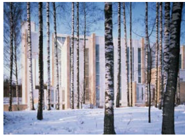
Myyrmäki Church, in Vantaa (near Helsinki); 1980-84, photo by Arno de la Chapelle
